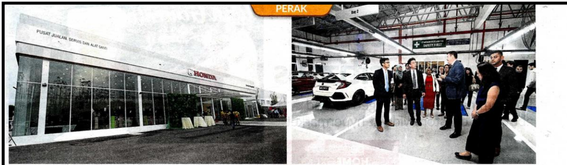
The Ban Hoe Seng Auto 3S Centre in Klebang, Ipoh, is the first building in Perak to receive the Green Building Index Gold certification. — Photos: RONNIE CHIN/The Star
